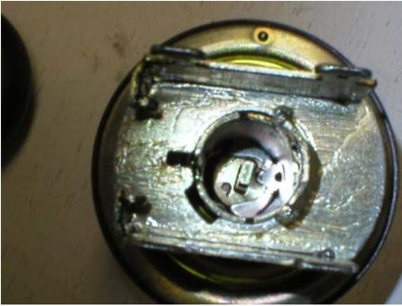
Finish turning the tailpiece until it is about 90 degrees to the original position. NOTE I turned the lock around (I'm right Handed)
